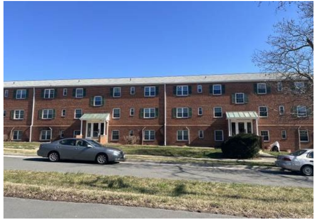
Greenwood Apartments north of Subject site (Excluded)
