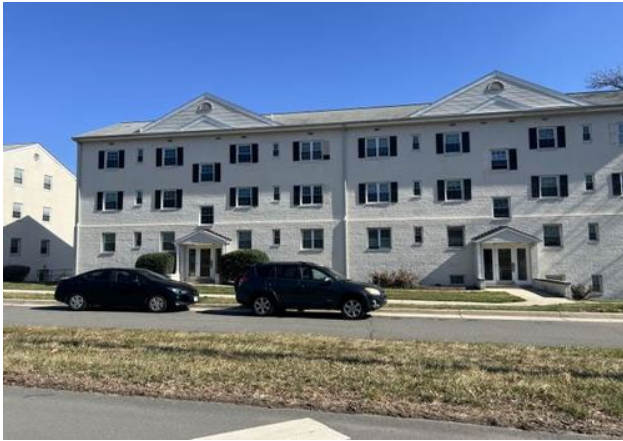
Greenwood Apartments north of Subject site (Excluded)
