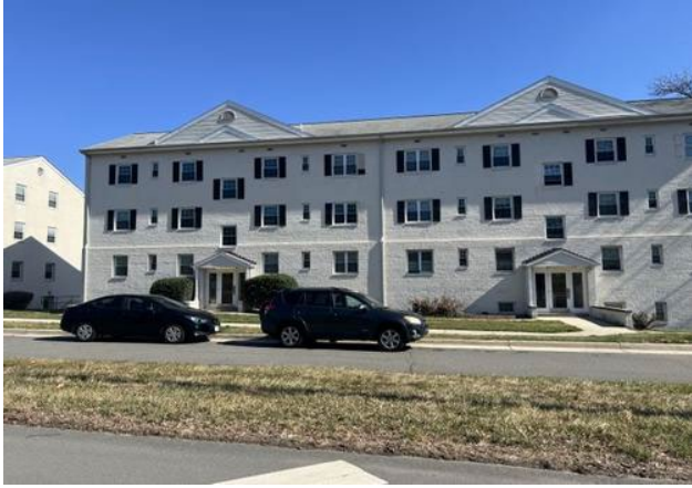
Greenwood Apartments north of Subject site (Excluded)
