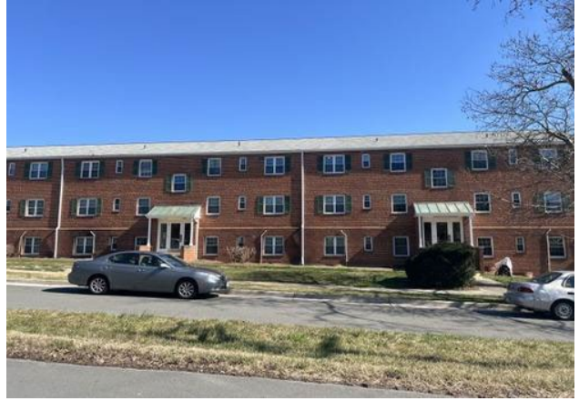
Greenwood Apartments north of Subject site (Excluded)
