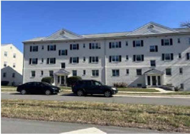
Greenwood Apartments north of Subject site (Excluded)
