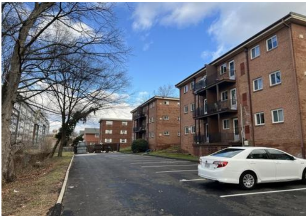
Existing building and parking lot on Subject site
