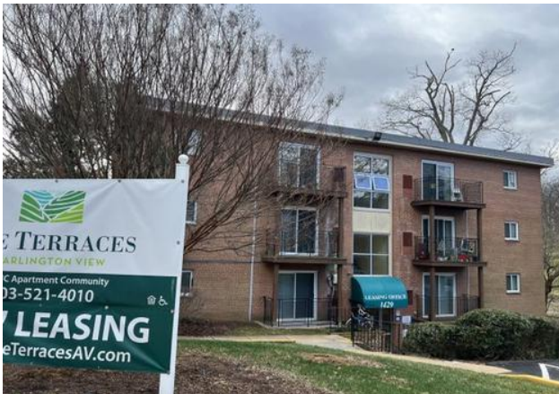
Existing building on Subject site
