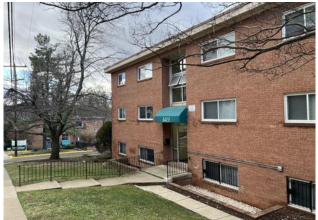
Existing building on Subject site
