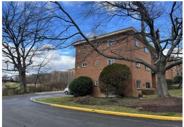
Existing building and driveway on Subject site
