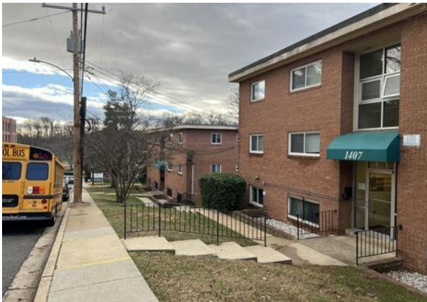
Existing building on Subject site
