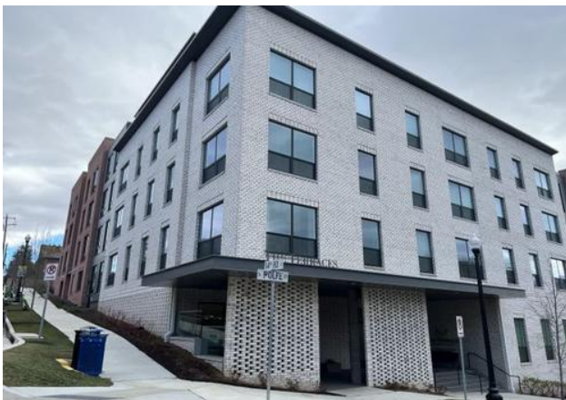
Arlington View Terrace East (comparable) directly east of Subject site
