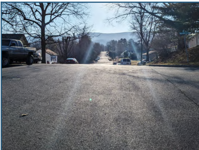
Streetscape: East view along 3rd Street
