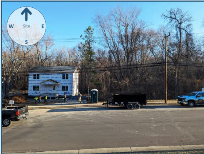
North view from site
