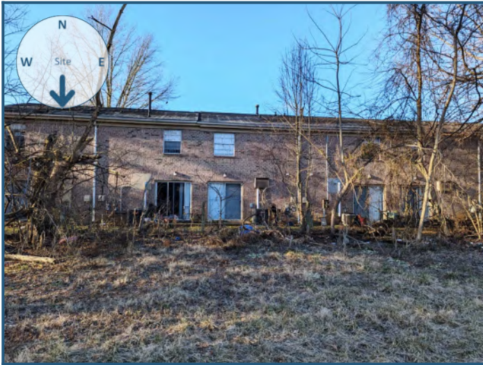
South view from site
