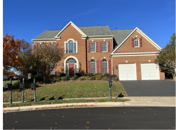
Typical single-family home south of the Subject
