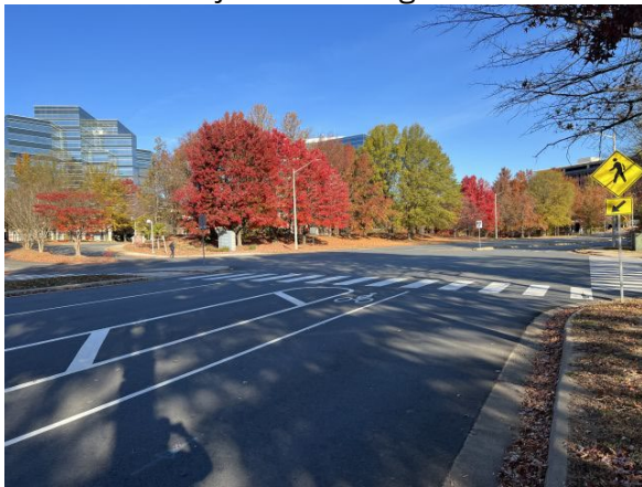
View along Government Center Parkway facing north
