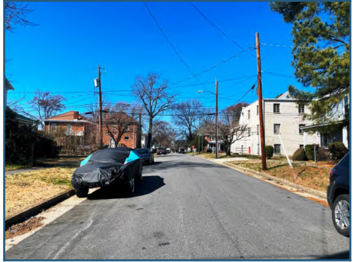
Streetscape: West view of Custer Street
