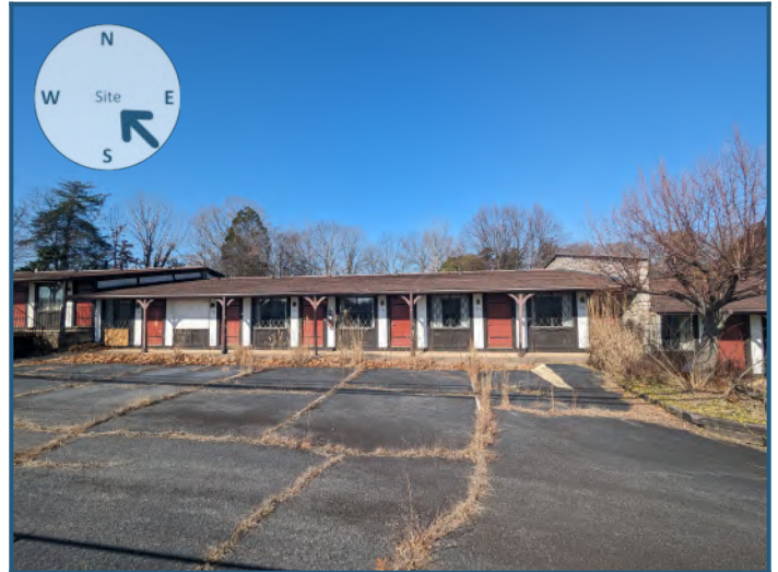
View of site from the southeast
