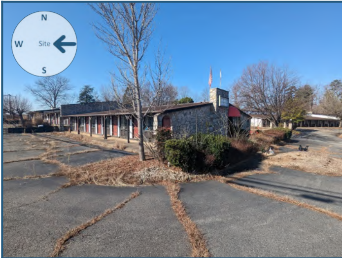
View of site from the east
