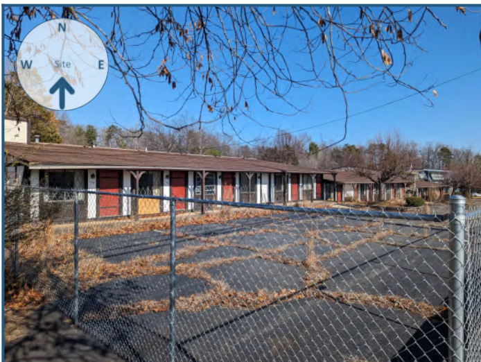
View of site from the south
