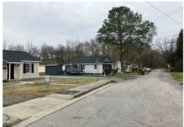
View facing south along Evans Street
