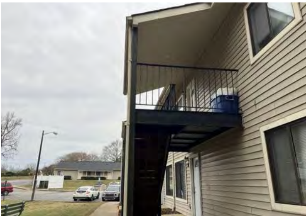
Typical Subject staircase
