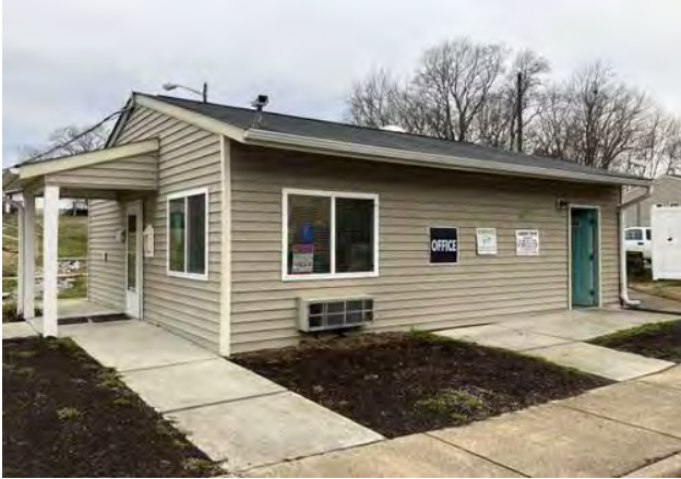
Subject leasing office
