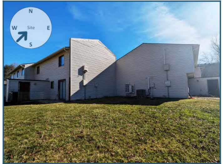
View of site from the southwest
