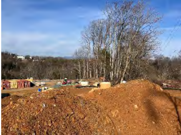
View of Subject site and site for Millers Rest Phase II
