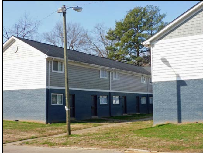
View across Lynhaven Ave (Lynhaven Apartments)
