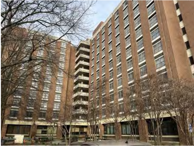
Existing multifamily development on Subject site (to be razed)
