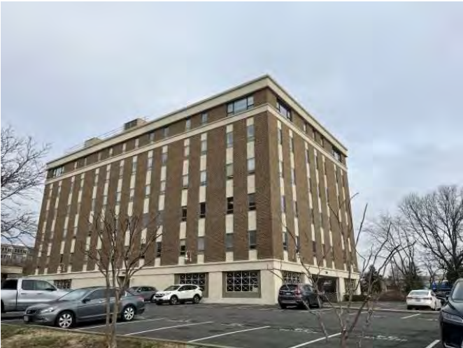
Office building north of the Subject site
