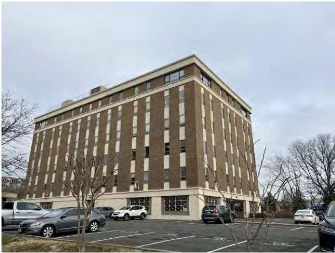
Office building north of the Subject site
