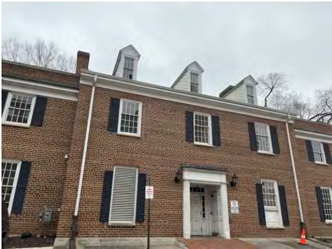
Office building on Subject site (to be razed)
