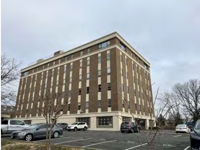
Office building north of the Subject site
