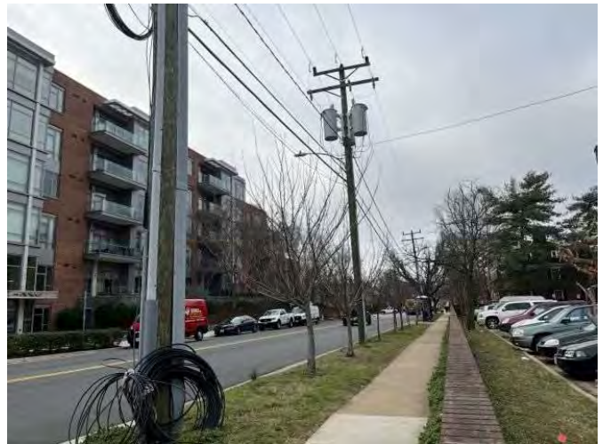
View south along North Fairfax Street
