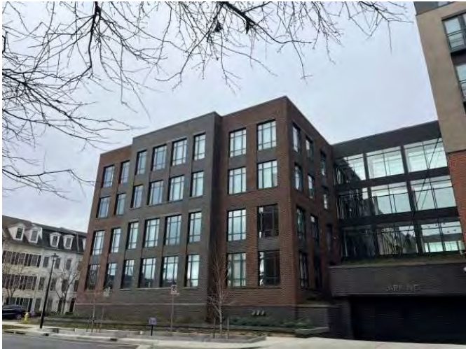
Alexan Florence (included) west of the Subject site
