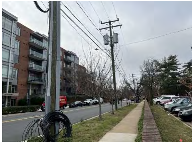
View south along North Fairfax Street
