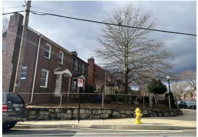
Rowhomes east of Subject site
