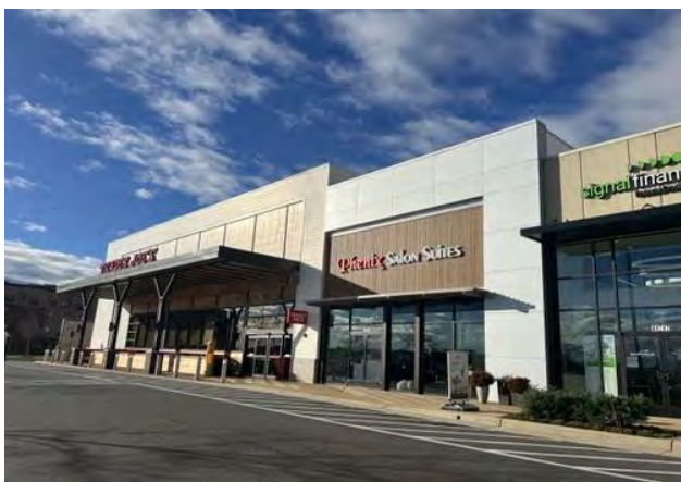
Typical commercial/retail uses in Subject's neighborhood
