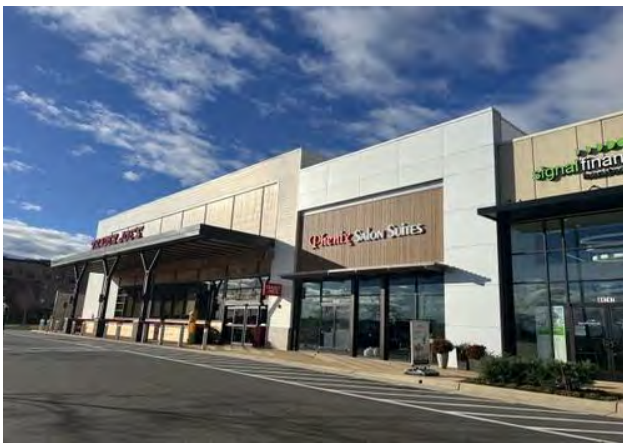
Typical commercial/retail uses in Subject's neighborhood
