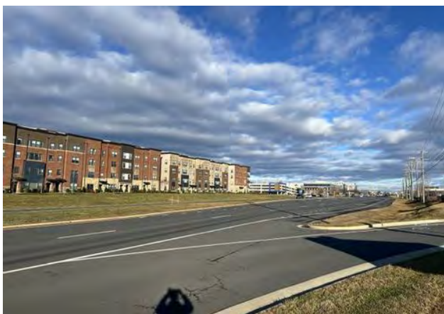
View north along Loudoun County Pkwy.
