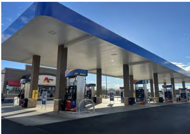
Nearby gas station
