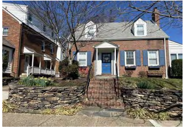
Nearby Single-family Home in Average Condition
