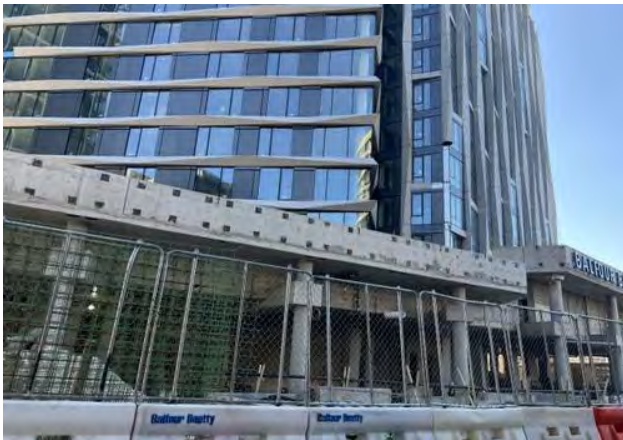
Nearby New Construction on 20th Street
