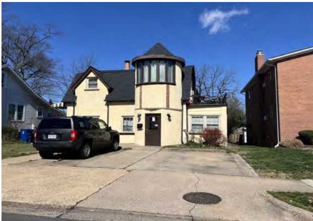
Nearby Single-family Home in Average Condition
