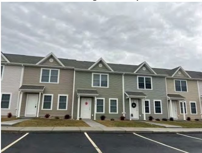
Millwood Townhomes (owner-occupied) south of the Subject site
