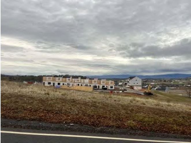
Single-family homes under construction north of the Subject site
