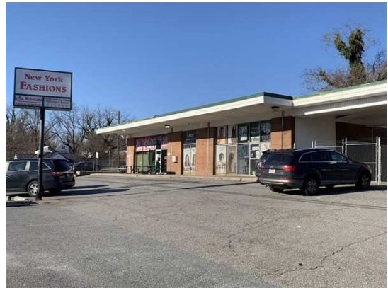
Retail center west of site
