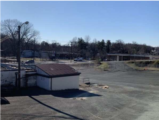
View of site facing west from SW 5 th Street
