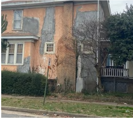
Residential property west of site as seen from Woodcliff Ave
