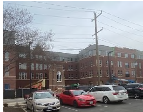
Highland Terrace Apartments under construction north of site
