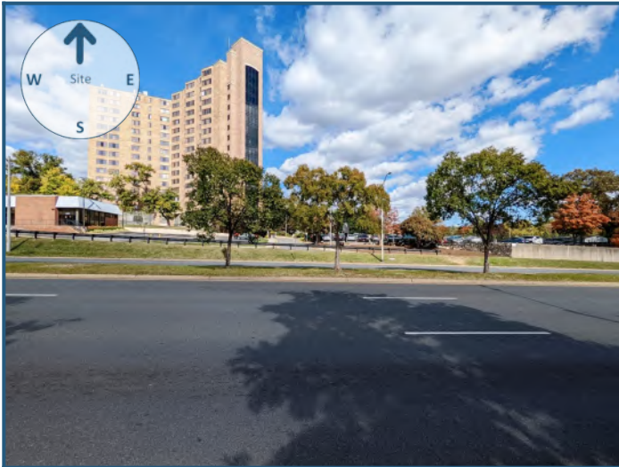
North view from site
