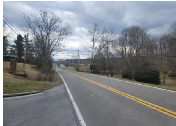
Looking South From Entrance
