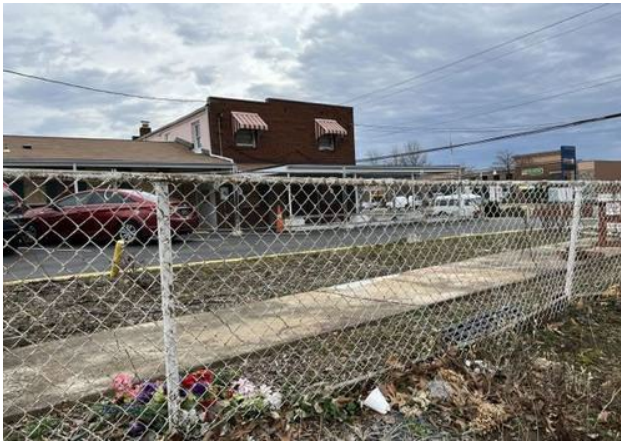
Subject site (existing building to be demolished)
