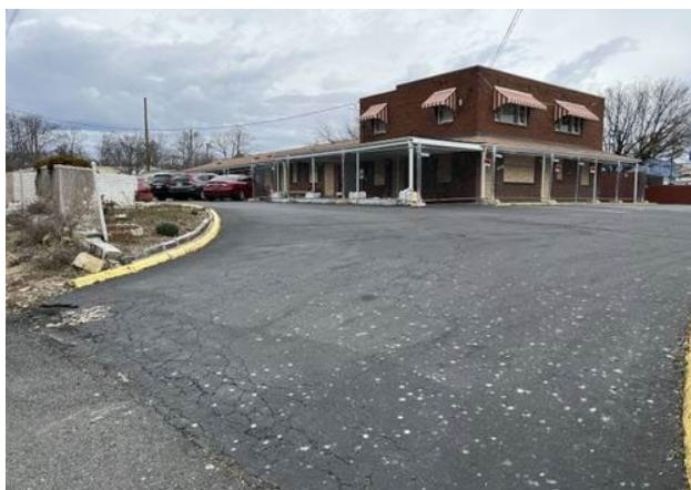
Subject site (existing building to be demolished)
