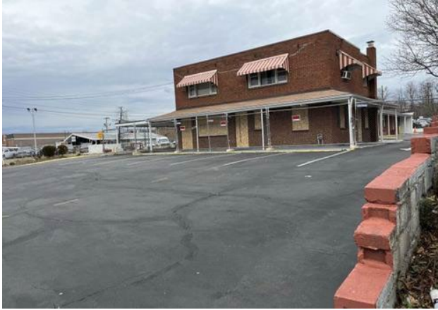
Subject site (existing building to be demolished)
