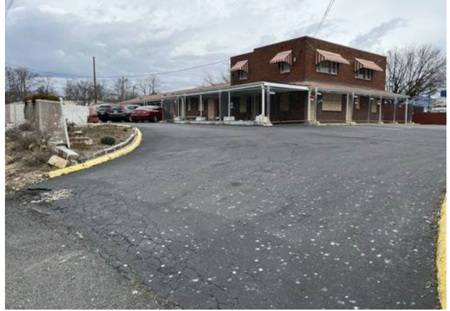
Subject site (existing building to be demolished)
