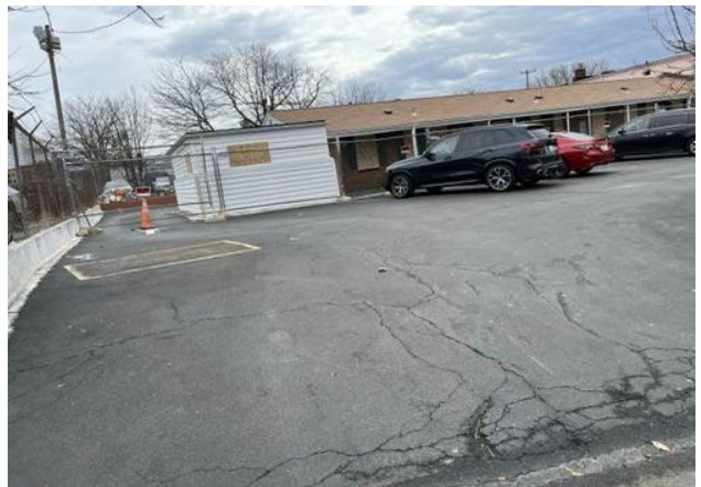
Subject site (existing building to be demolished)
