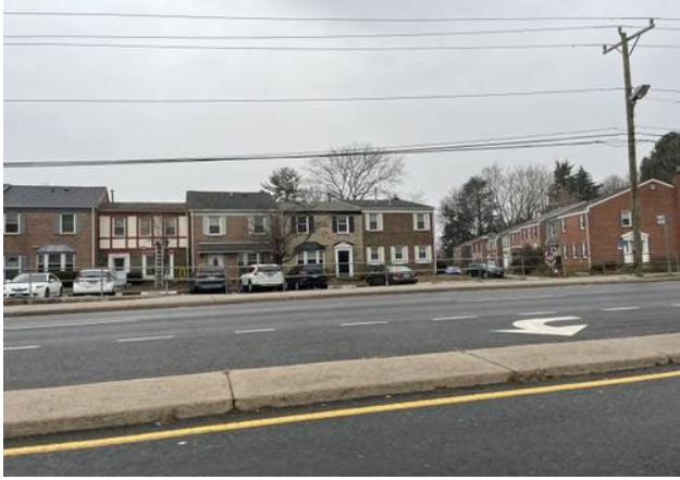
Single-family homes in Subject neighborhood
