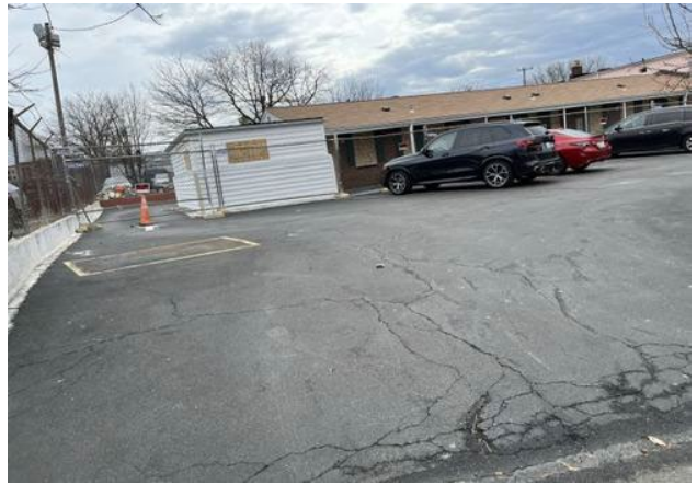
Subject site (existing building to be demolished)
