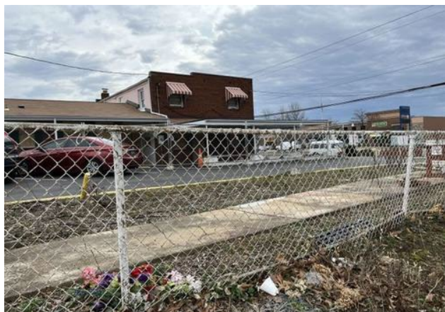
Subject site (existing building to be demolished)
