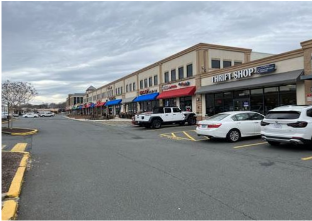
Commercial south of Subject site
