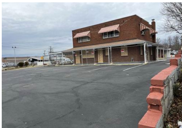
Subject site (existing building to be demolished)
