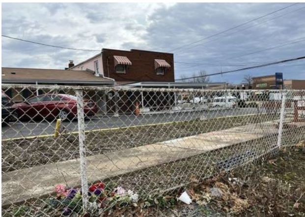
Subject site (existing building to be demolished)
