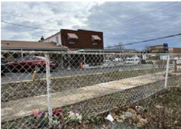
Subject site (existing building to be demolished)
