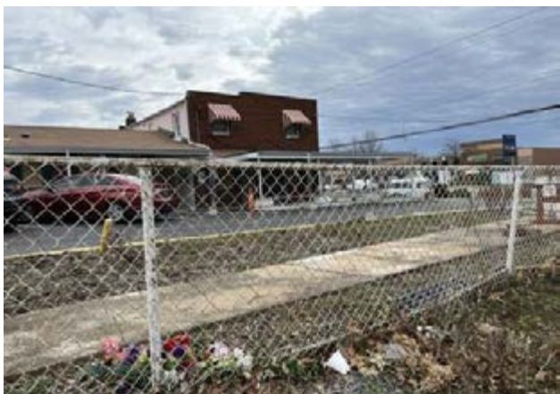
Subject site (existing building to be demolished)
