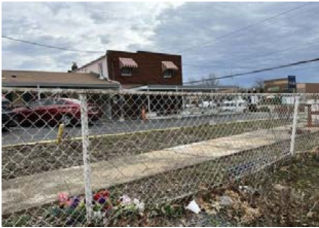
Subject site (existing building to be demolished)
