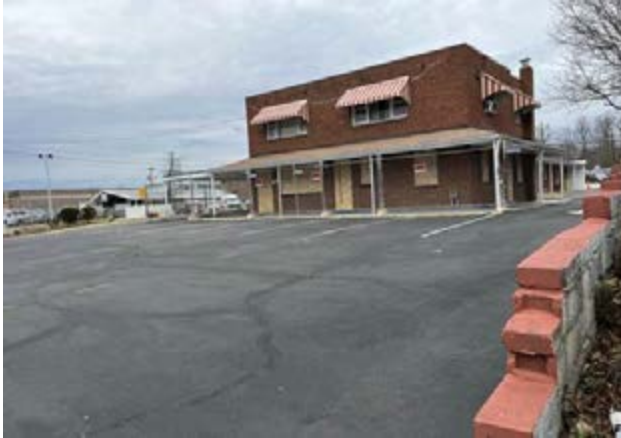
Subject site (existing building to be demolished)
