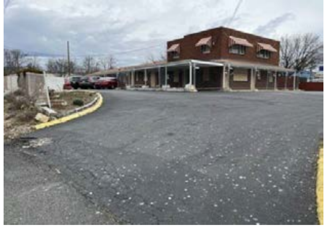
Subject site (existing building to be demolished)
