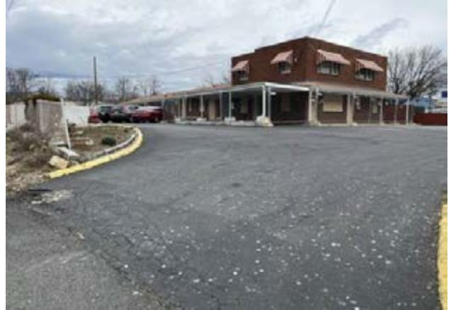
Subject site (existing building to be demolished)
