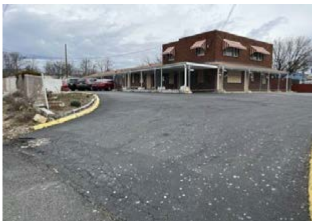
Subject site (existing building to be demolished)
