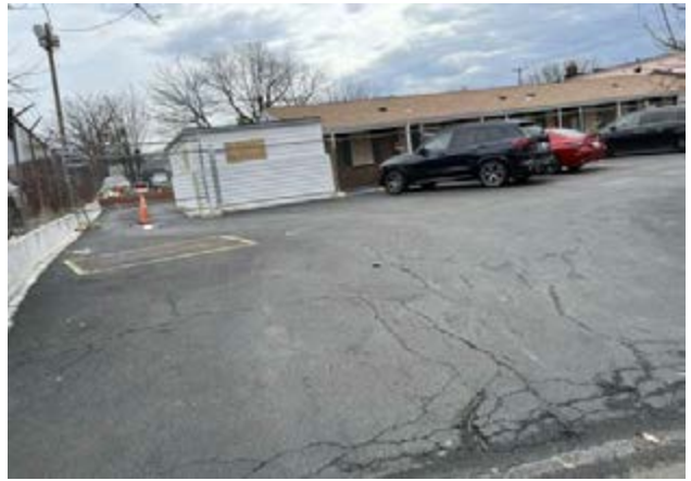
Subject site (existing building to be demolished)
