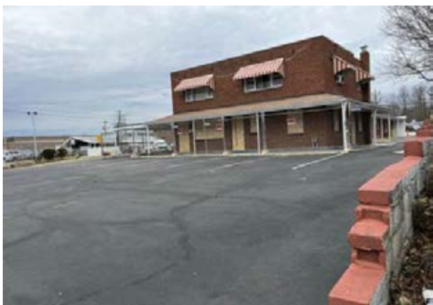
Subject site (existing building to be demolished)
