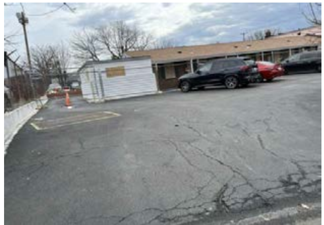
Subject site (existing building to be demolished)
