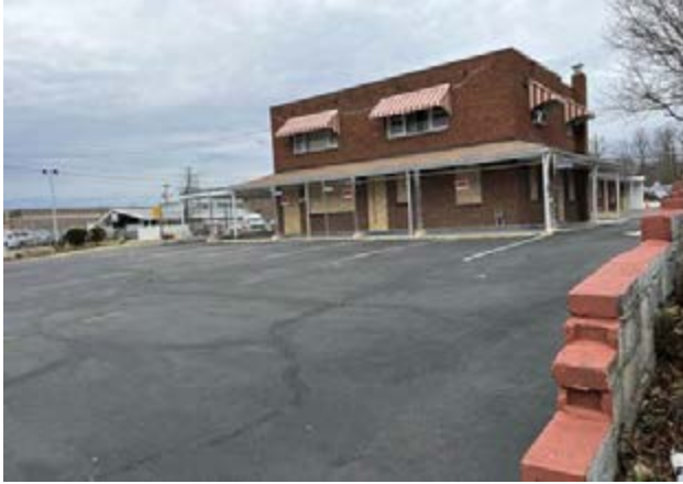
Subject site (existing building to be demolished)
