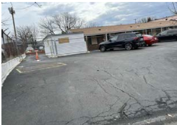
Subject site (existing building to be demolished)
