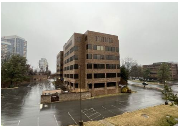
Office building adjacent to Subject site
