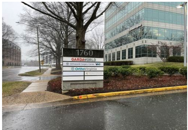
Office building adjacent to Subject site
