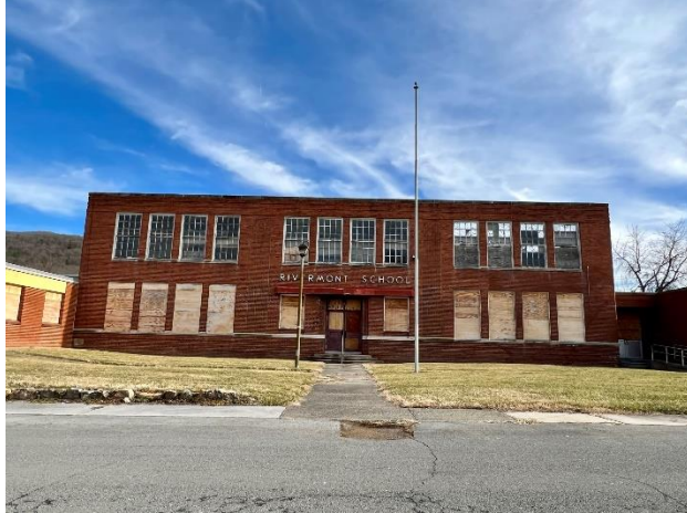
Front View of School Building from N Rockbridge Avenue
