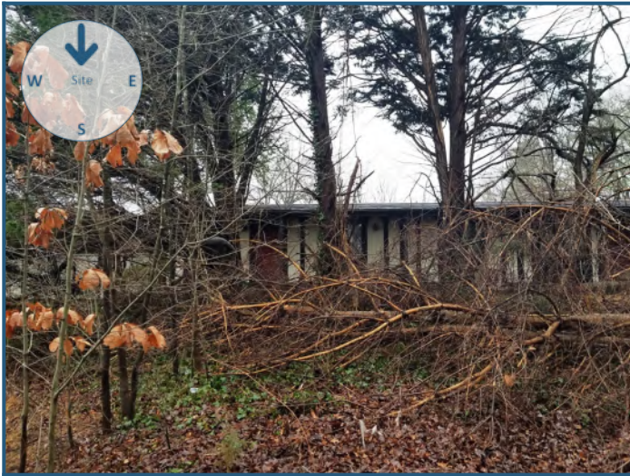
View of site from the north
