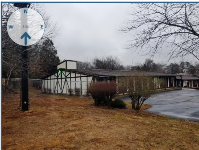
View of site from the south
