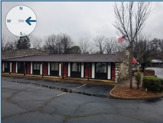
View of site from the east
