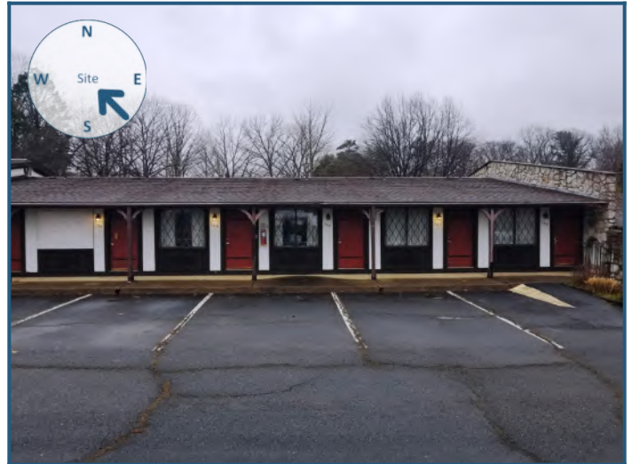
View of site from the southeast
