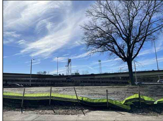
Interstate 264 south of site
