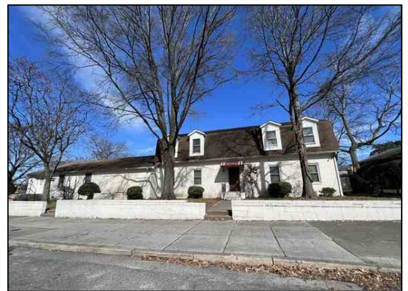
View from the center of the site facing east
