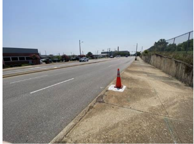
View south along Commerce Road
