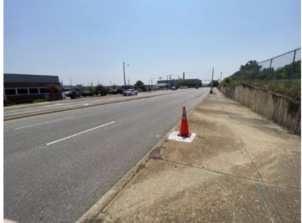
View south along Commerce Road
