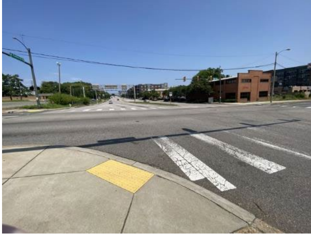
View north along Commerce Road
