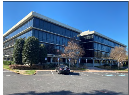
Site facing northwest from southeast corner of subject
