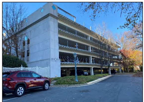
Parking garage, immediately west of site
