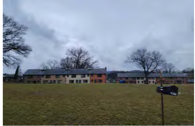
Looking South From Entrance
