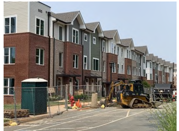
Construction of Phase I looking North along 6 th St SE
