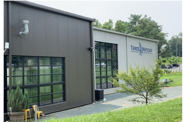
Looking southwest from site - Three Notched Brewery
