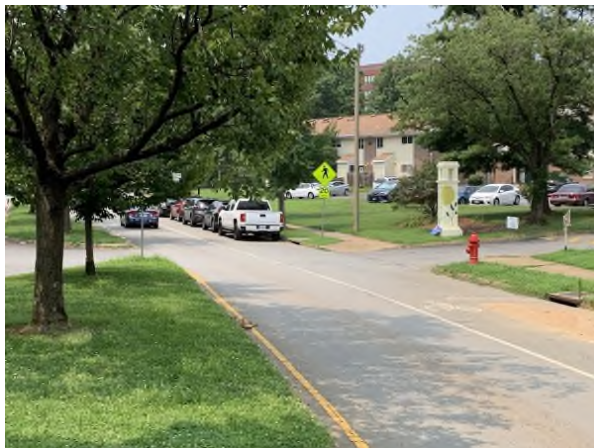
Looking west along Monticello Ave (site on right)
