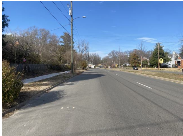
View north along Westover Hills Boulevard
