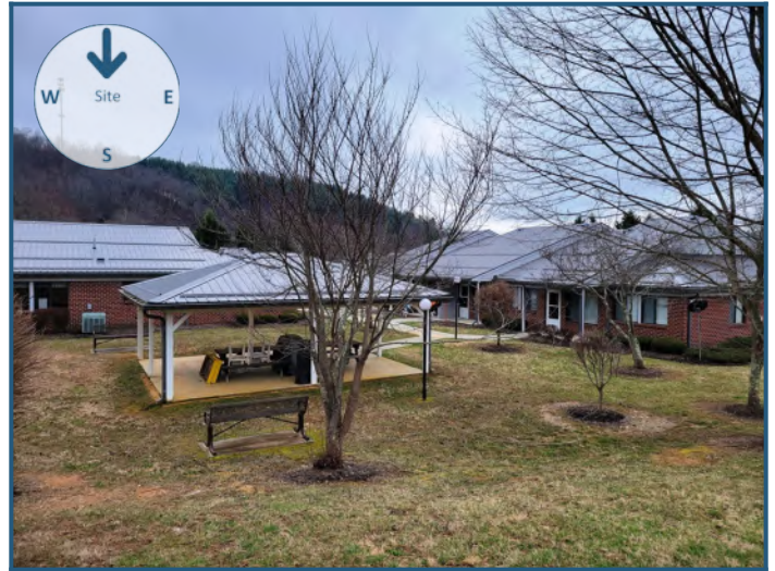
View of site from the north
