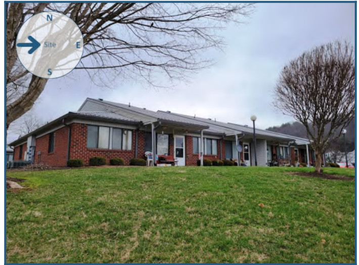
View of site from the west
