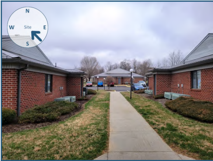
View of site from the southeast
