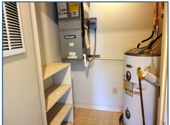
One-Bedroom (Storage/Water Tank Area)
