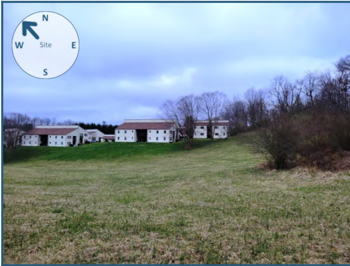
Northwest view from site
