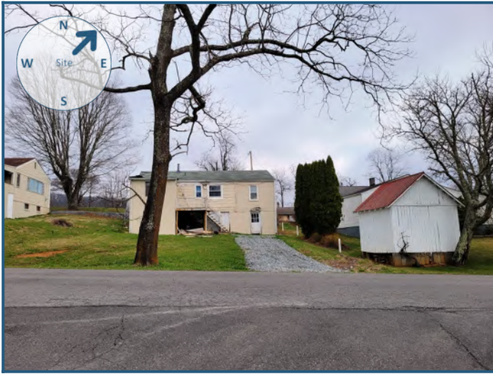
Northeast view from site
