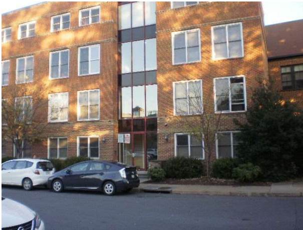
Norcross Station new construction building
