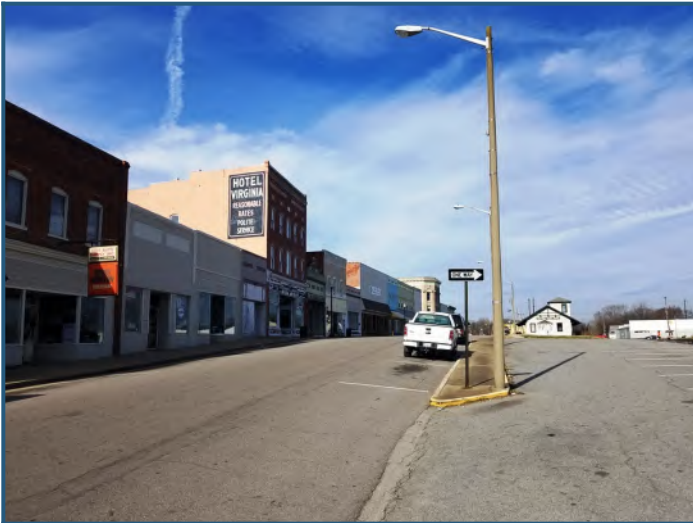
Streetscape: North view of Halifax Street
