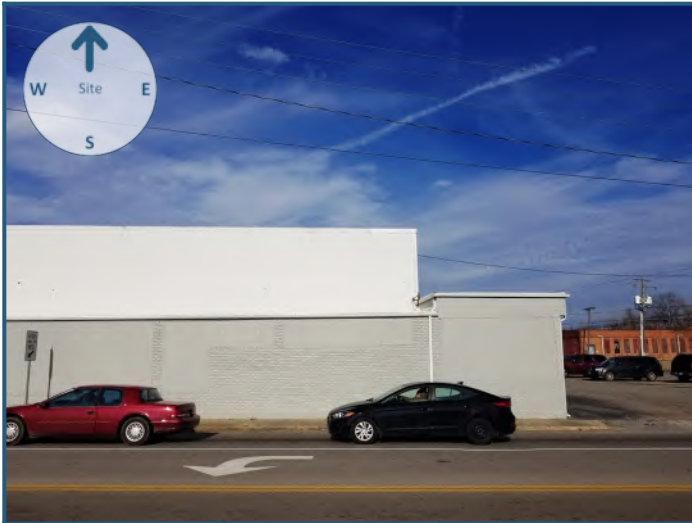
North view from site
