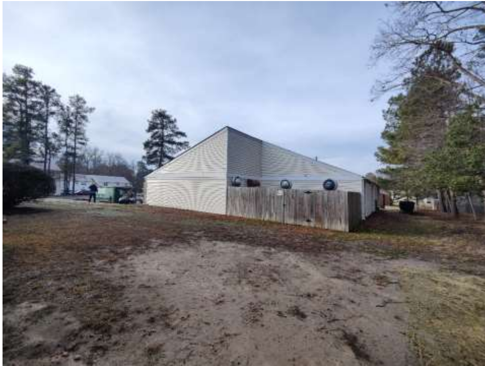
View to the North
