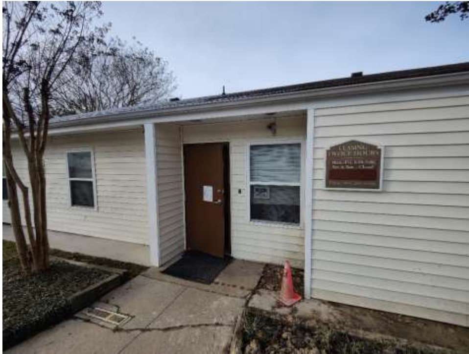
View of Office Building
