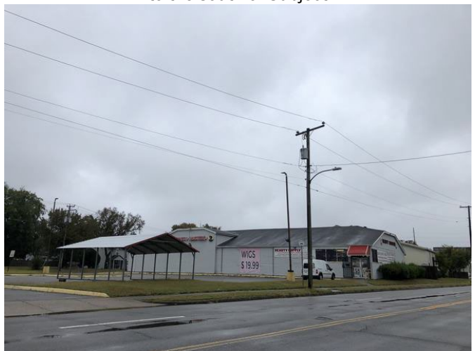
Retail building along Deep Creek Boulevard, west of Frederick Boulevard, several blocks south of Subject
