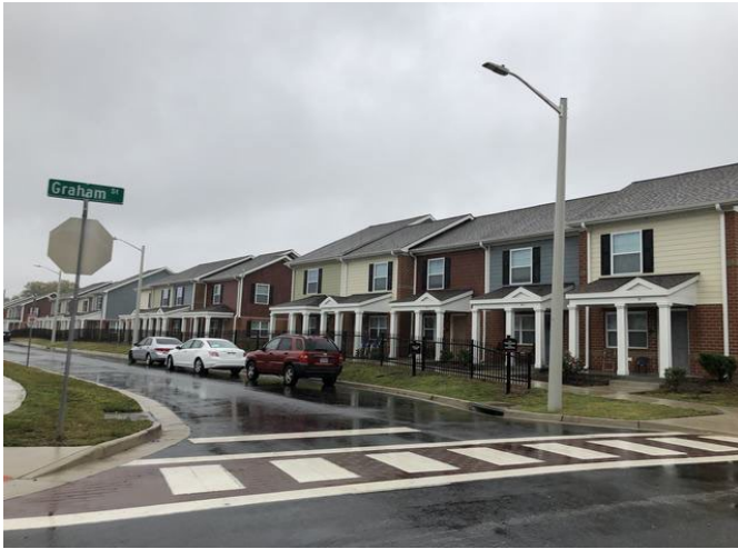
Lexington Place adjacent to the south of Subject site
