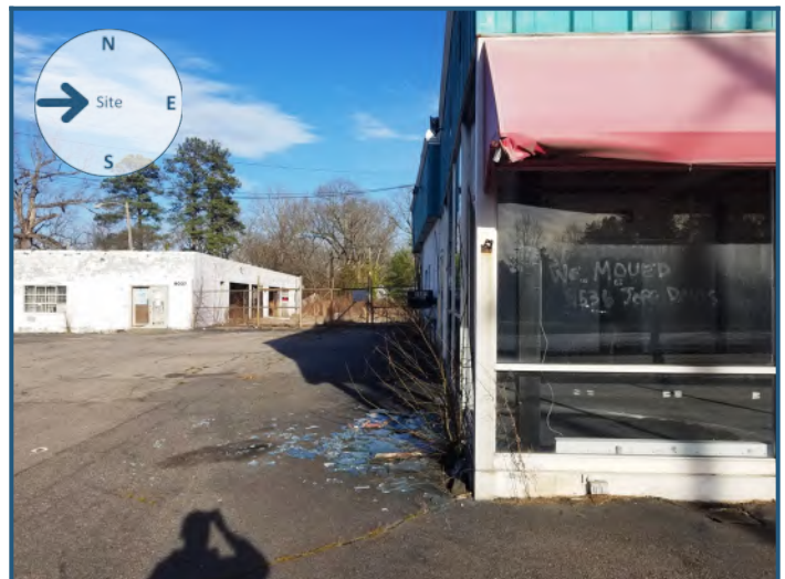
View of site from the west
