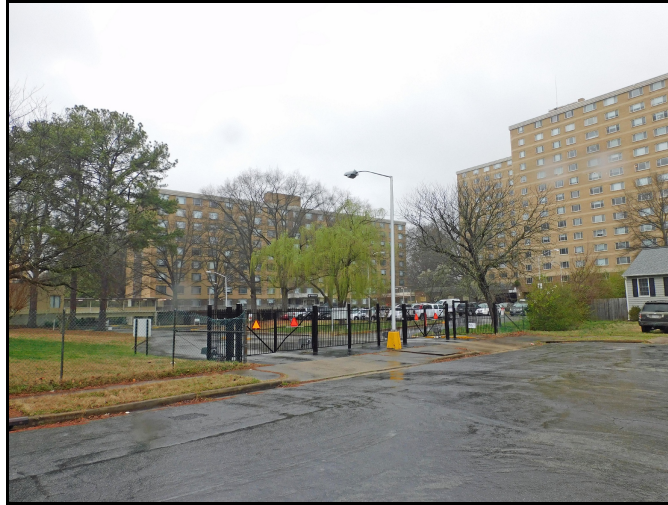
View of gate at Hill Monument and Rosedale
