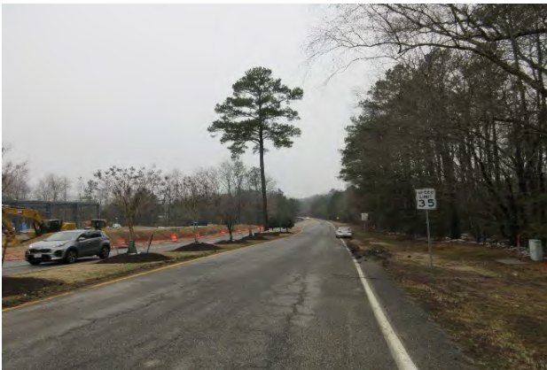
Looking East From Entrance
