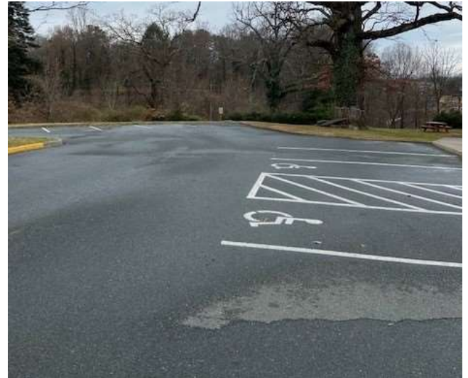
Looking south across site
