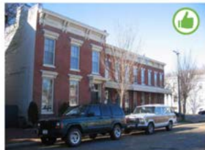
Exterior Material — Brick
