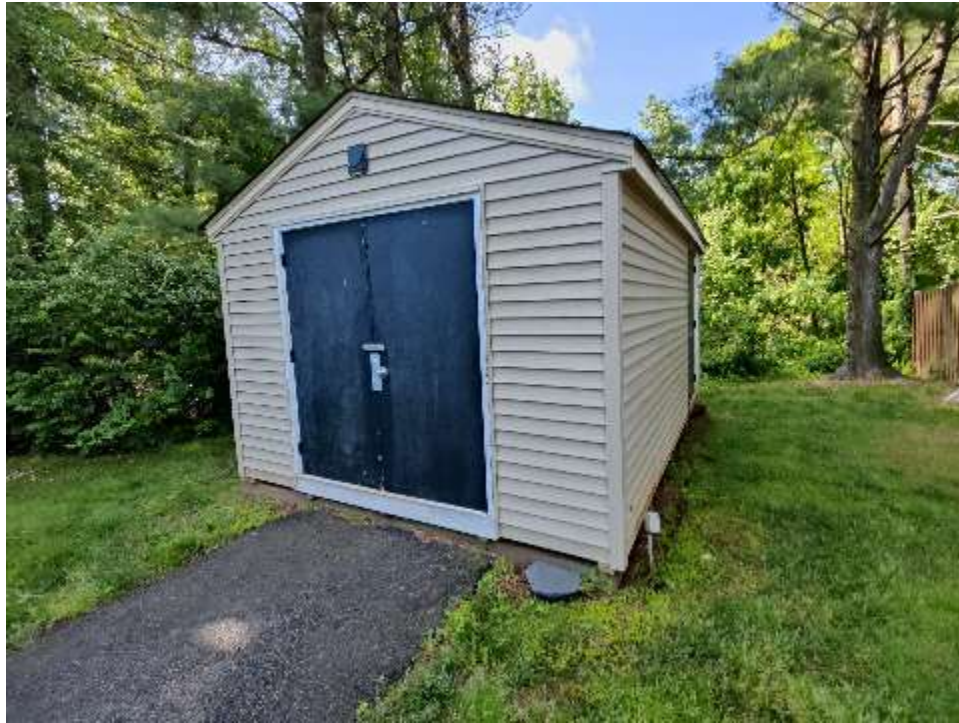
View of Maintenance Shed
