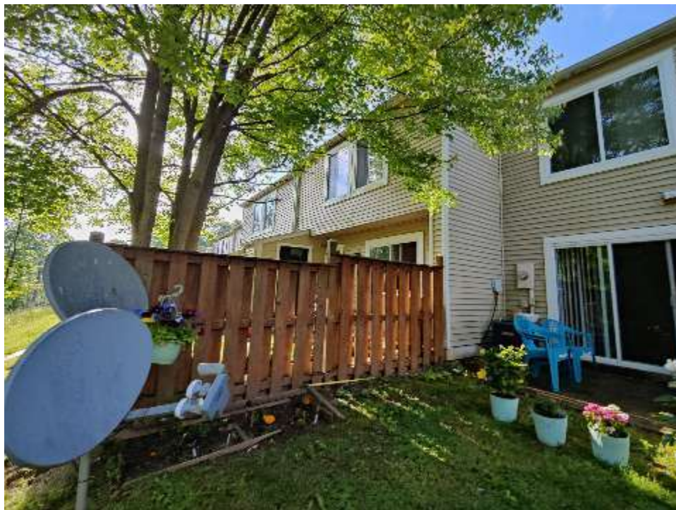
View of Typical Patio
