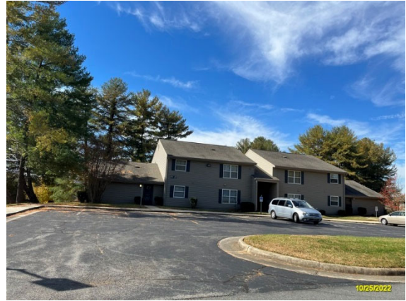
Typical Subject Building
