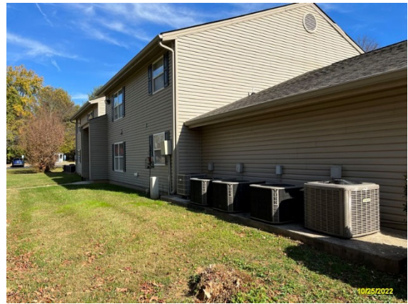
Typical Subject Building (Rear)
