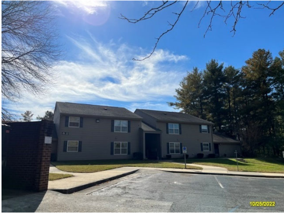
Typical Subject Building
