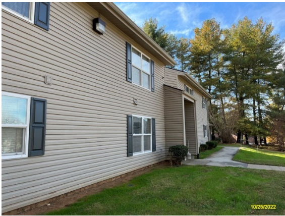
Typical Subject Building
