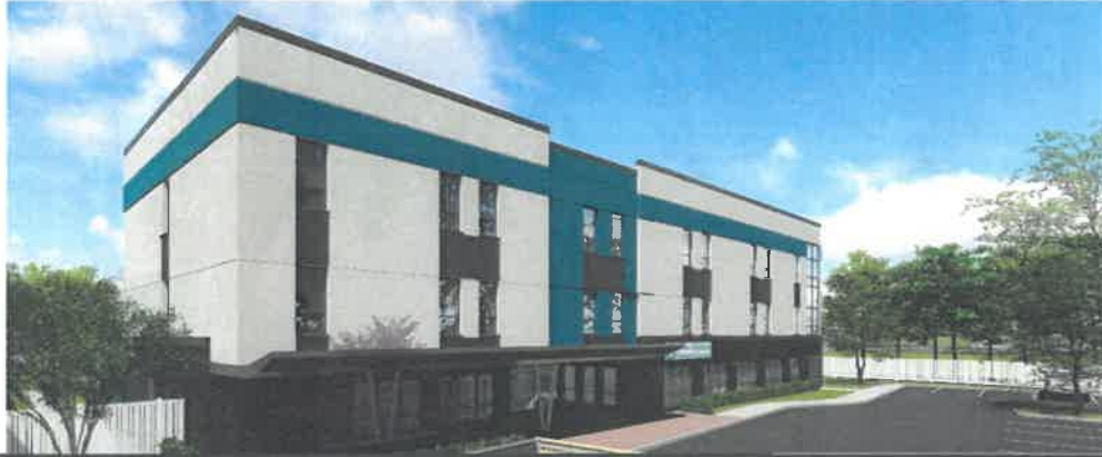
Virginia Beach Facade Welcoming Canopy and Offices
