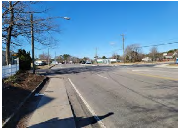
Looking West From Entrance
