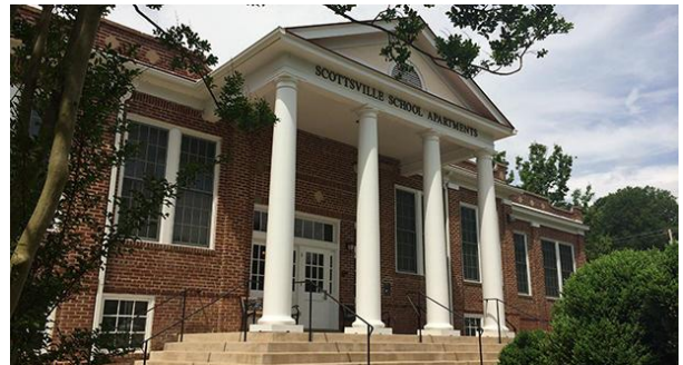
Scottsville School Apartments
