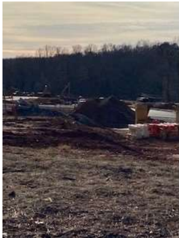
Construction site for SF homes south of 4% parcel
