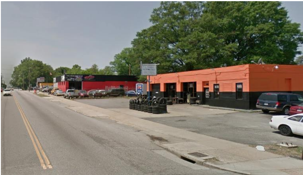
Commercial Business Along E 36 th Street
