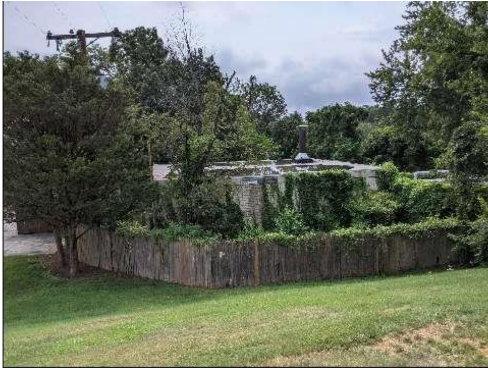
View of Mechanical Building
