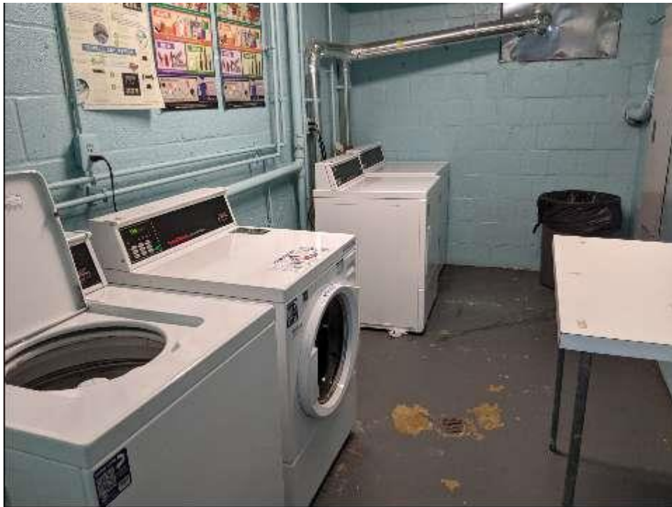
View of Laundry Facility
