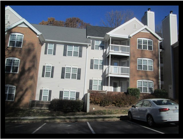
7) EAVES FAIRFAX CITY
