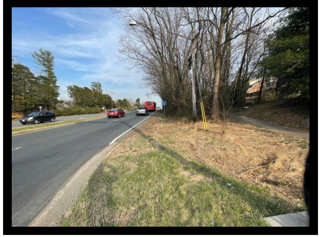
FACING EAST FROM NORTHWEST CORNER OF THE SITE
