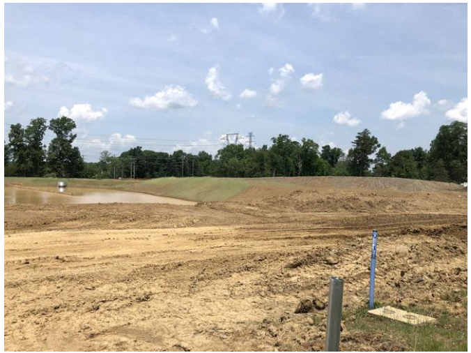
View of storm water pond to the north of Subject site
