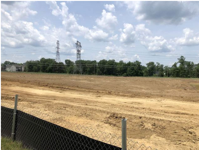
Alternative view of Subject site
