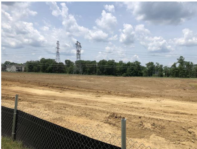
Alternative view of Subject site
