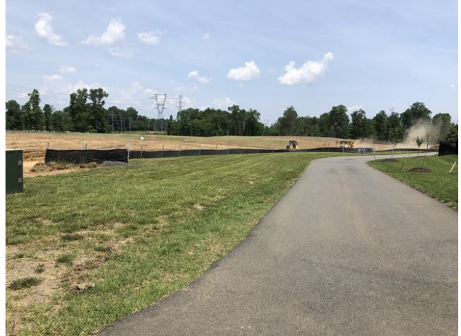
Subject site looking northwest from Calderwood Lane
