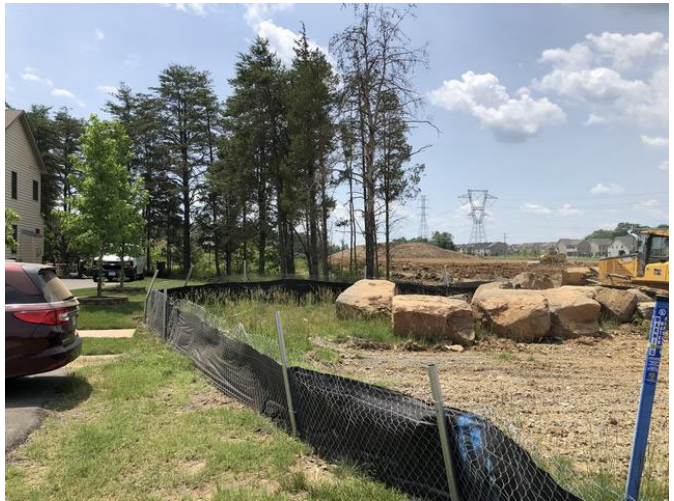
View to the south of Subject site
