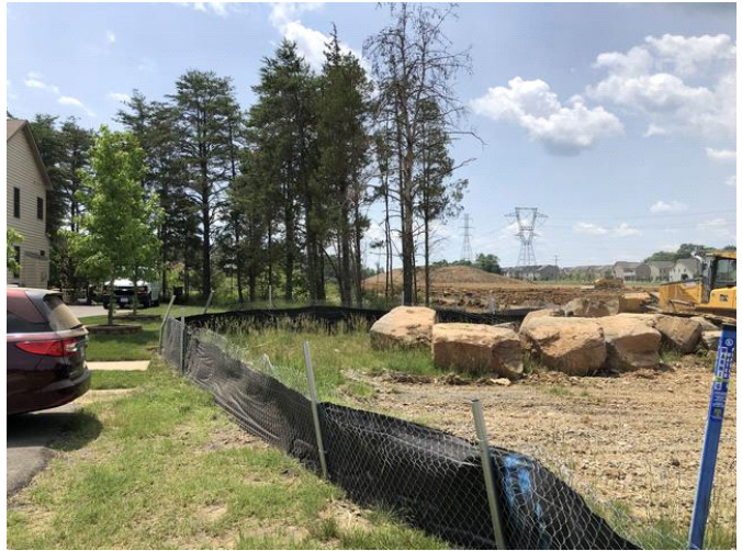
View to the south of Subject site
