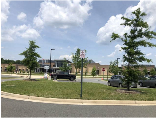
Independence High School south of Subject site
